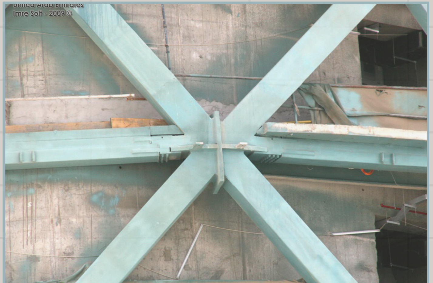
Concrete and steel skeleton
